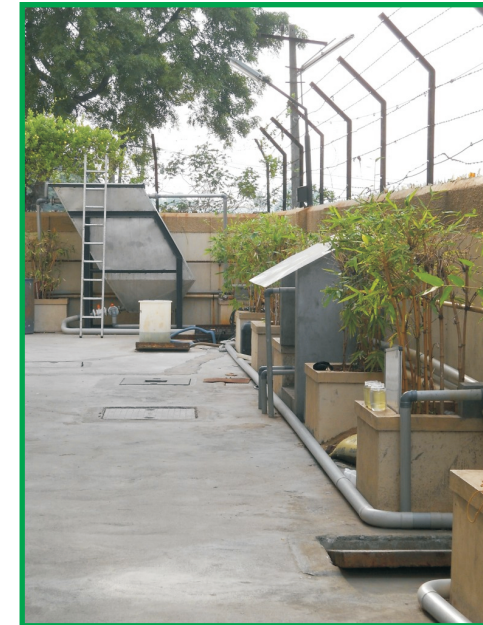
Underground Advanced SBR
